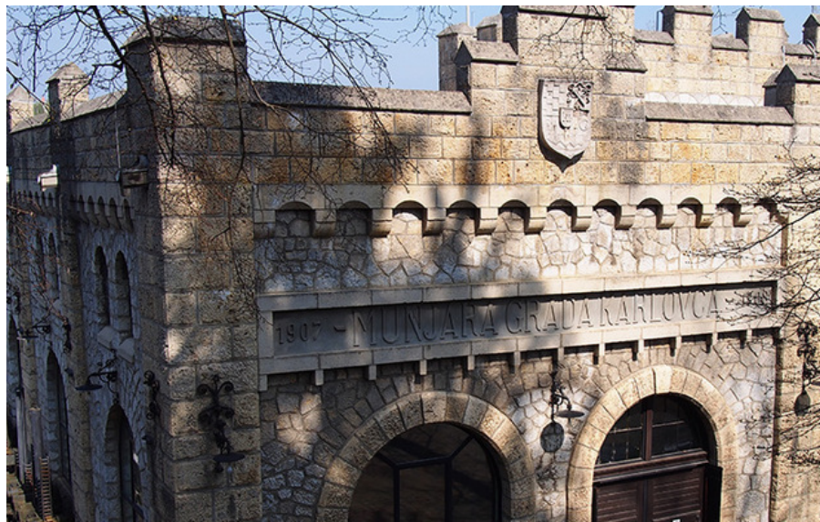
Karlovac munjara in the town of Ozalj (viewed from the main entrance)
